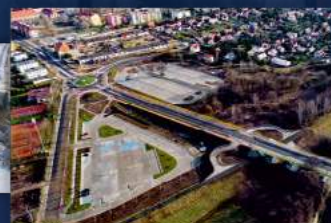
Renovation of the road Legnica, Poland
